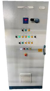
This panel is for the Fume Extraction and Scrubber unit. It powers the fan and allow for the Scrubber to operate automatically by monitoring the pH levels and dosing via a pump as and when required. This reduces the risk of error by an operator, and saves time.
