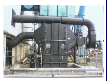
We design fume extraction to suit your requirements, this is determined by the tank dimensions, the quantity of tanks to be extracted, the type of chemical and the operating temperature. We can supply the complete system including the side hoods, manifold, stack, fan and a scrubber if required.
