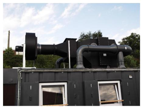
This customer was limited for space so the process line was inside a shipping container. We placed the extraction on top of it to make use of the space.
